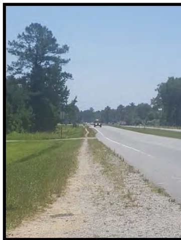
Figure 3-7: Worn dirt path adjacent to US Highway 17
