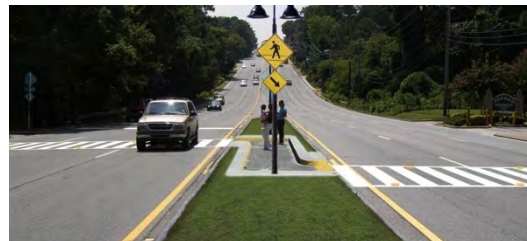
Staggered median crossing (Credit: Marcel Schmaedick)
