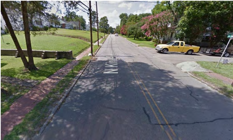
Figure 4-26: King Street & Spring Street Looking Northwest – Before (Source: Google Maps).
