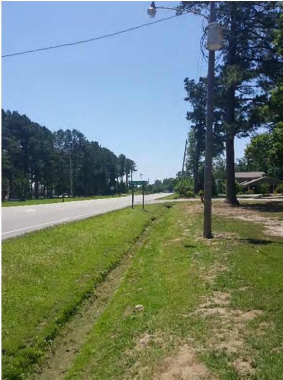
Figure 4-2: Cooper Hill Road Looking Northeast – Before (Source: HCP).
