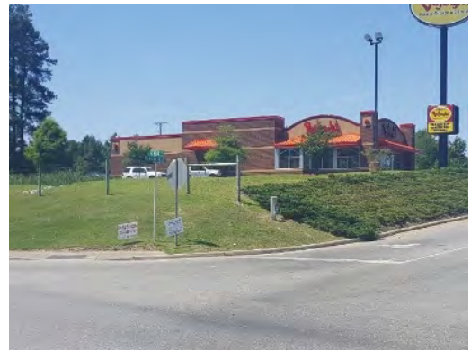
Figure 4-17: King Street Intersection near Bojangles Restaurant (Source: HCP).
