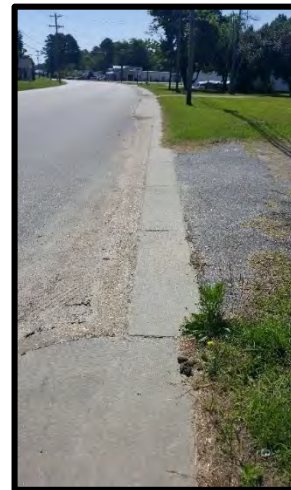
Figure 3-5: Deficient Sidewalk Infrastructure (S. King Street)
