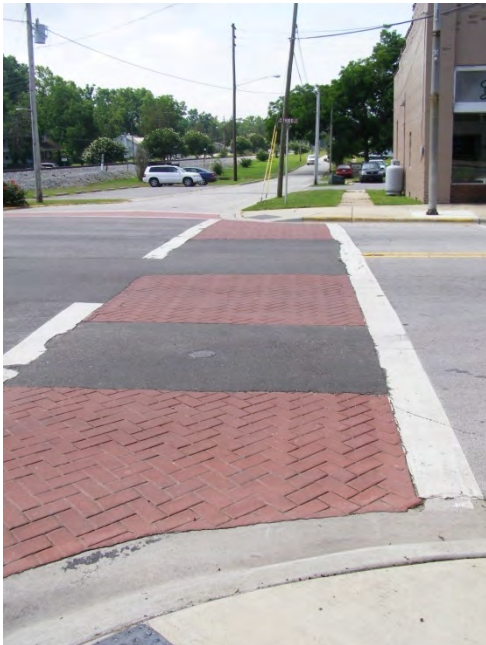
Decorative crosswalk treatments, as shown here in Ayden, NC made of distinctive materials can become uneven over time.
